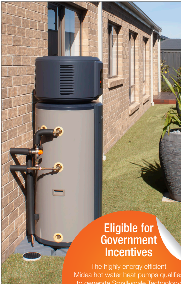
170L Installed Unit
