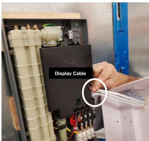
Figure 1: Removing Display Cable
